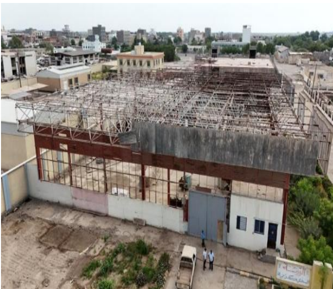
The Irrigation Gates Workshop, Dar Sa'ad district, Aden, assessed for rehabilitation | Photo credit: UNDP
