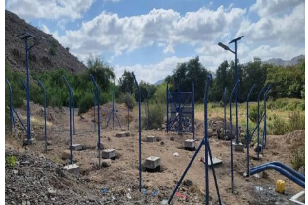
Early stage of constructing solar panel mounting structures in Al-Mosaymer district | Photo credit: UNDP
