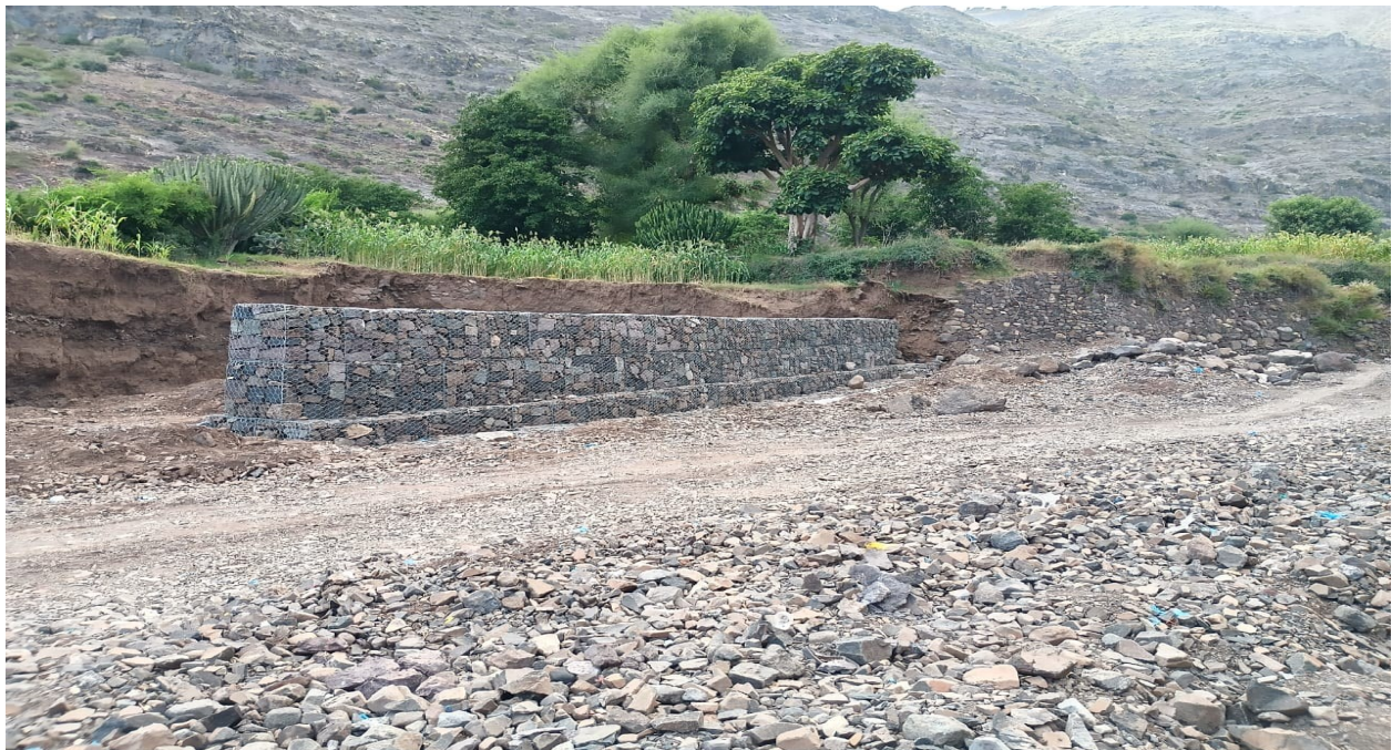
A flood gabion wall in Al-Mawaset district | Photo credit: UNDP.
