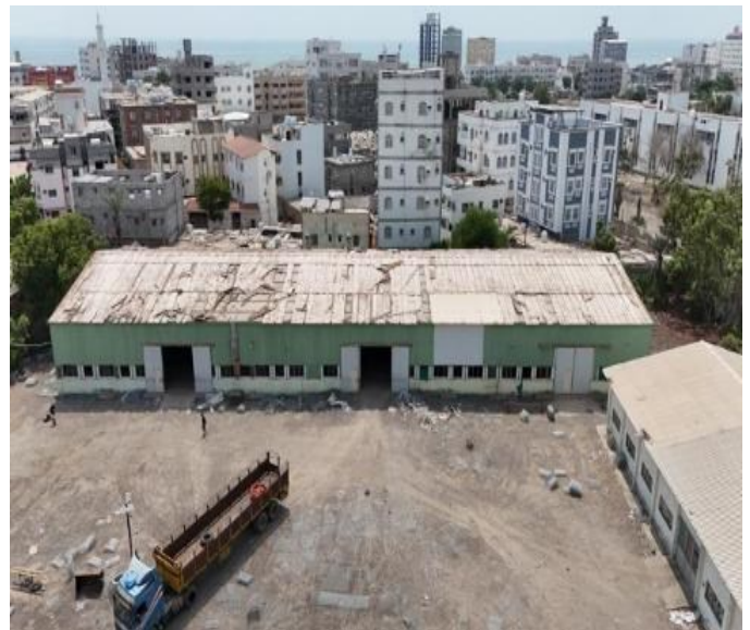
The Gabion Mesh Factory, Khormaksar district, Aden, before rehabilitation | Photo credit: UNDP
