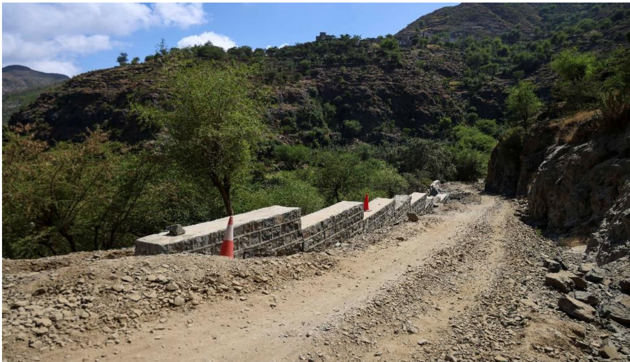
A rural road in Al-Mawaset, Taiz, targeted for stone pavement. The photos also show retaining wall recently constructed by the project illustrating how the project's integrated interventions reinforce one another | Photo credit: UNDP
