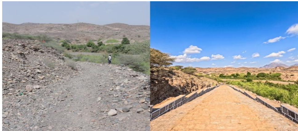
Al-Tanan 2 road- before & after rehabilitation, Al-Mosaymer district | Photo credit: UNDP
