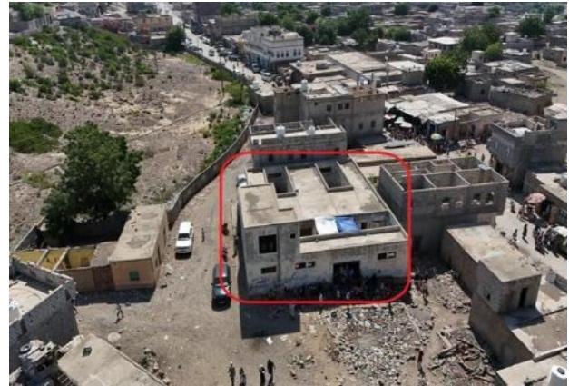
Market building before the rehabilitation in Al-Mosaymer district | Photo credit: UNDP
