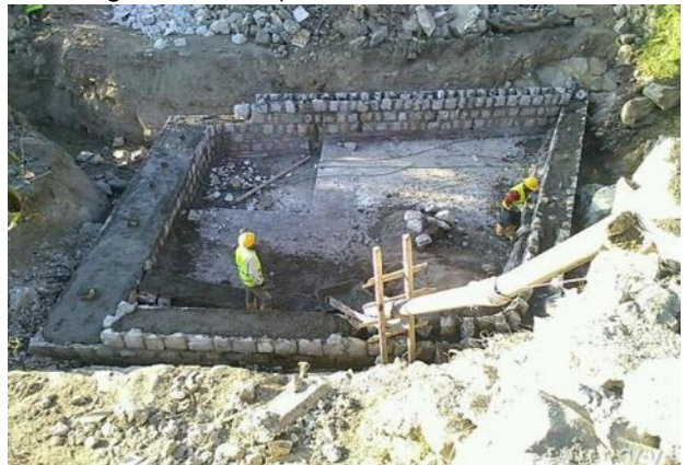
During construction of Al-Hoayd Al-Sofla Pond in Al-Selw District | Photo credit: UNDP
