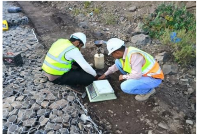
Soil compaction testing (>95 percent) following backfilling and compaction works behind the gabion walls – Taiz | Photo credit: UNDP
