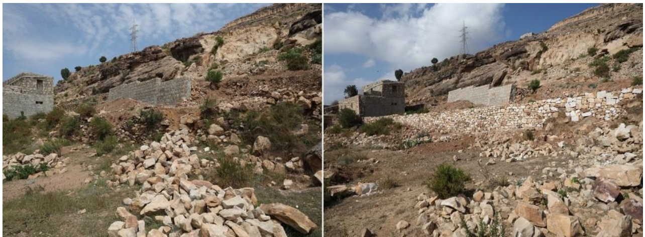
An agricultural terrace in Al-Selw district before and after rehabilitation | Photo credit: UNDP
