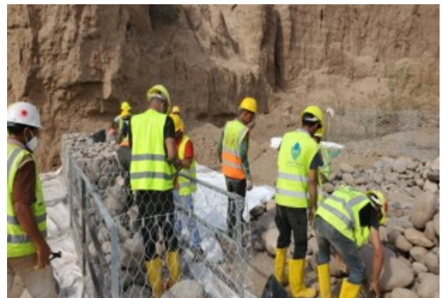
PPE compliance by workers during Package 1 implementation- Tuban | Photo credit: UNDP
